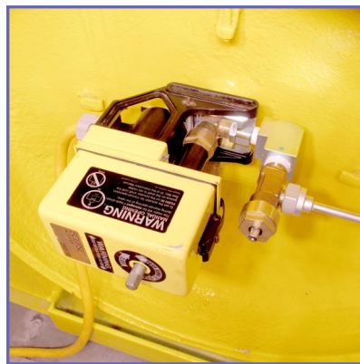
IV-830 with emergency shutoff actuator on a ton container with flexible connector.
